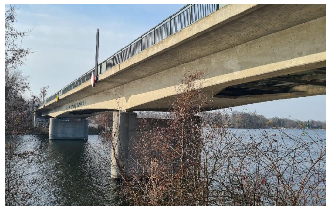
Figure 9. Baumgarten Bridge near Potsdam.
