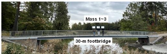
Figure 3. Experimental damage cases.
