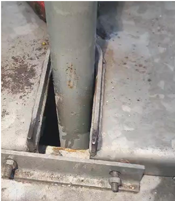
Figure 17. Contact of the hanger bar and cover plate
