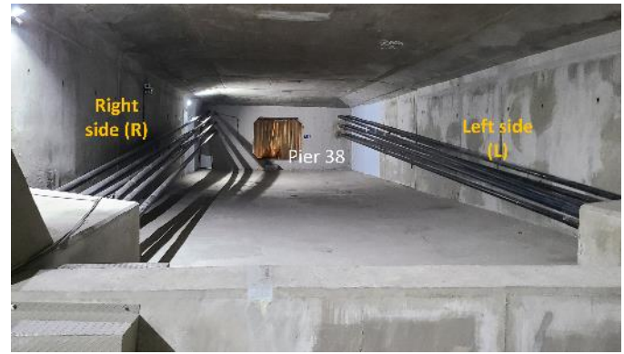
Figure 5. PSC box girder of test bridge
