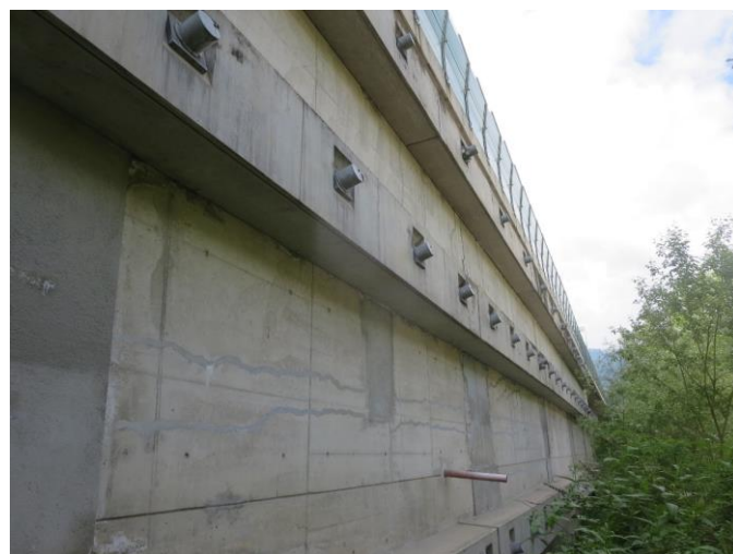
Figure 2. Pre-stressed anchors used for the remediation of a cantilever retaining wall.
