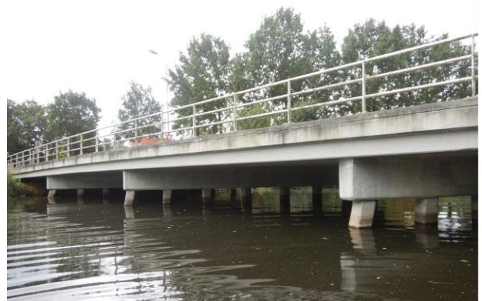
Figure 2-1 Side view of bridge (source: Google Streetview)
