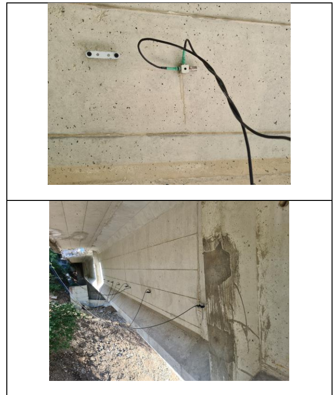
Figure 2. Sensor positions on La Patenda Bridge.
