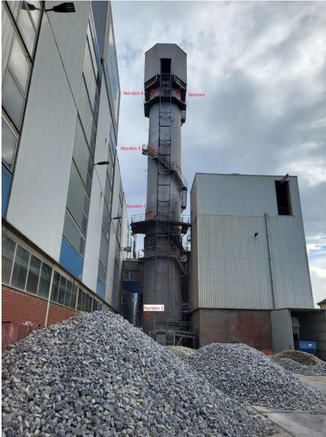
Figure 4: Sensor locations at the Südzucker Lime Kiln in Wabern/Germany
