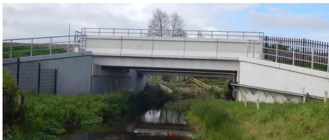
Figure 2. Bridge UB11, Staffordshire, U.K.
