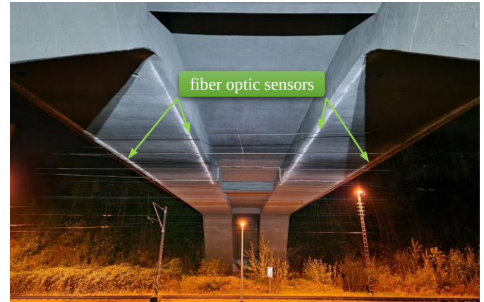
Figure 8. Layout of the sensors on the surface of hollow box
