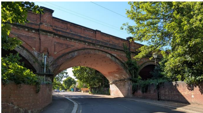
Figure 3. Bridge HDB-19, London, U.K.
