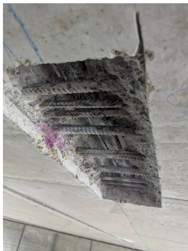
Figure 10. Sampling of prestressing wires from an existing road bridge for material testing (source: LS Brandenburg).
