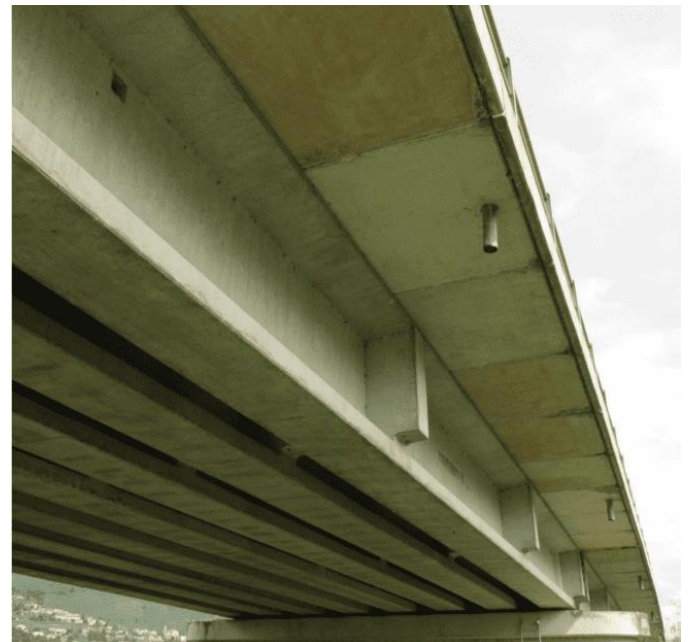
Figure 2: Intrados view of a typical span of the case study with the PRC beams.
