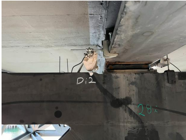
Figure 5 deck structure supported by the steel cross truss by elastomeric bearings.
