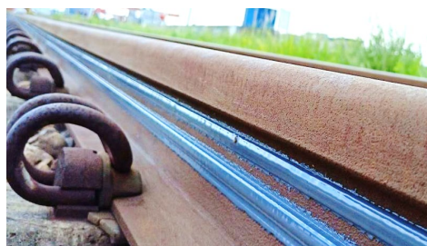
Figure 9. EpsilonFlats after test installation.
