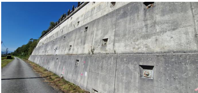
Figure 2: View of the anchor wall.
