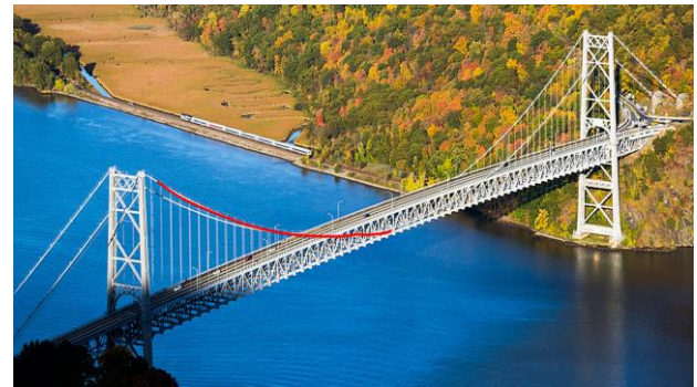
Figure 1: Schematic of the optical fiber (red line) installed at Bear Mountain bridge.
