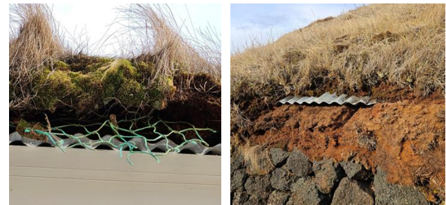
Figure 3: Examples of corrugated steel in turf roofs. A fishing net has also been added likely because the turf slides on the corrugated steel.
