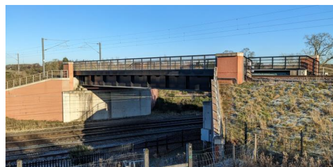
Figure 1: Bridge IB5, Staffordshire, U.K.
