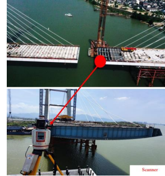
Figure 2. Tested bridge for closure in construction
