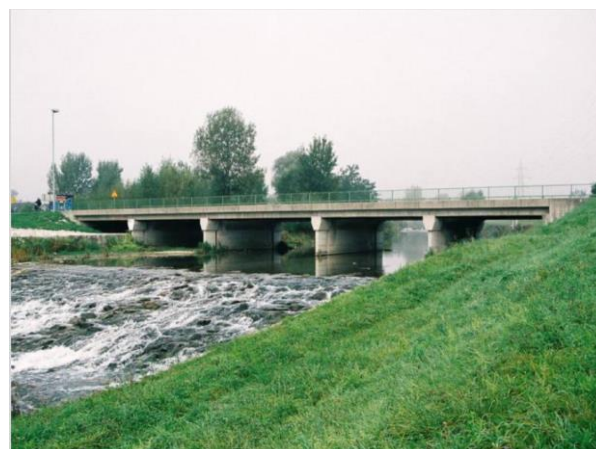
Figure 1. Existing bridge before the collapse (downstream).
