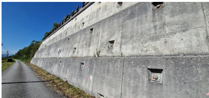
Figure 10. Segmented anchor wall.
