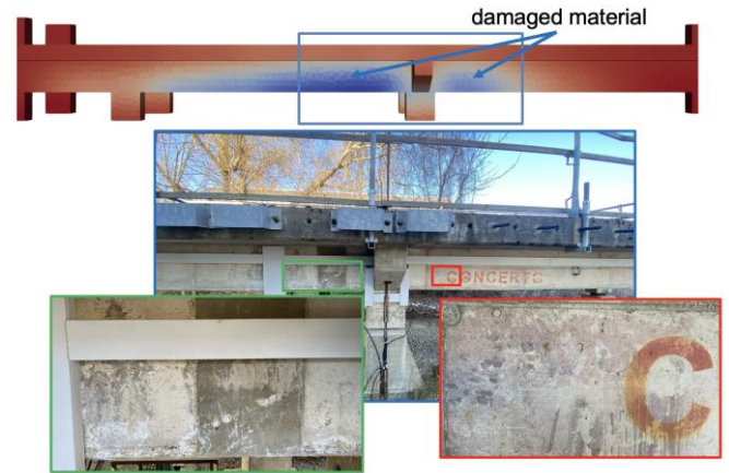
Figure 17. Top: Young's modulus of concrete. Bottom: Pictures of the current state of the bridge in the weakened regions.
