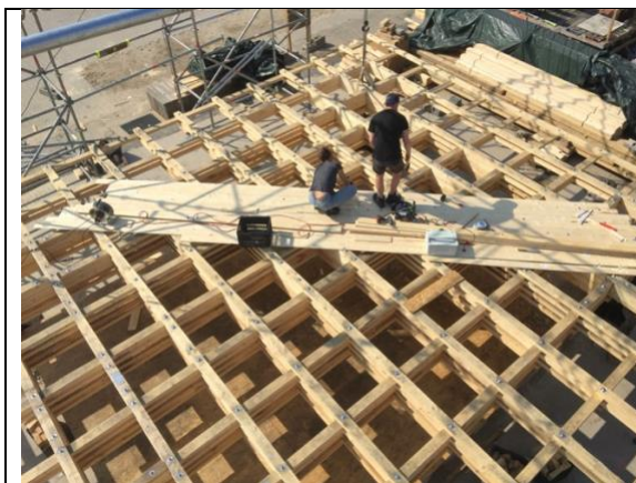
Figure 9. Infozentrale, installation roof construction, timber beam lattice grid
