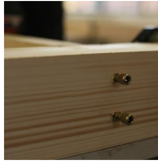
Figure 19. Screwed connection facade element
