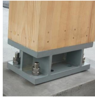
Figure 20. Bolted connection column - foundation
