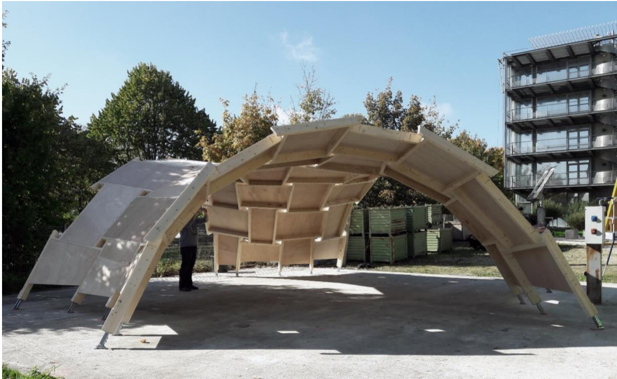
Figure 1. R2 Pavilion built with shell-nexorade hybrid structural system
