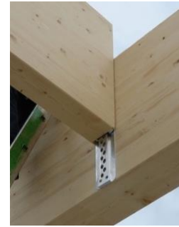
Figure 21. Reversible joist hanger (© Sherpa)
