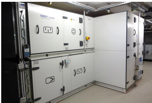
Figure 3: TROX X-CUBE ventilation system
