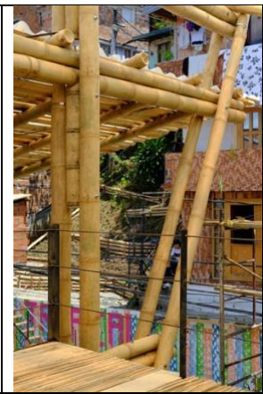
Figure 15. Taller Tropical Detail, frame corner
