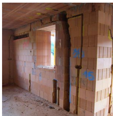
Figure 9. Drilling and chiselling work on the construction site for electrical installations and water pipes with popular tools [7].
