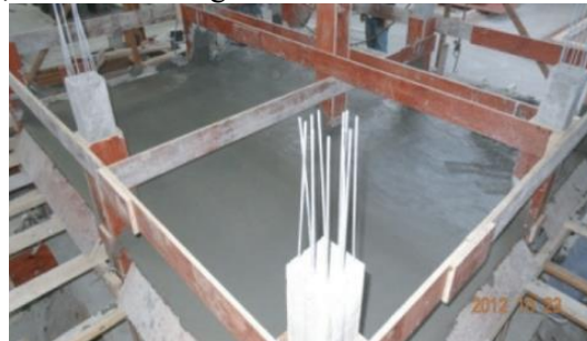
Figure 7. Casting joints and slabs.
