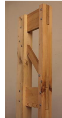
Figure 14. Framework stud, different sized batters, assembled centrally
