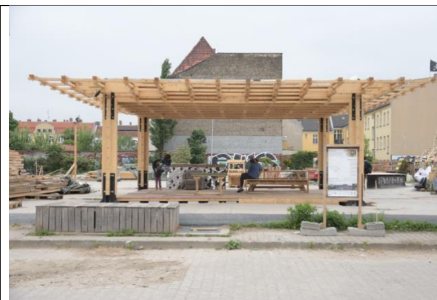
Figure 10. Infozentrale, raw construction, timber beam grillage, fixed columns
