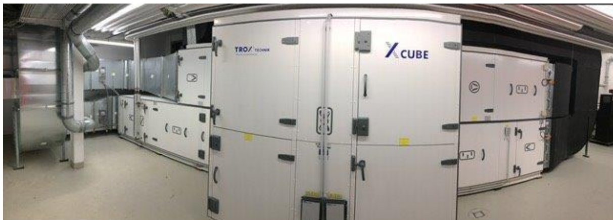
Figure 7: TROX X-CUBE ventilation unit
