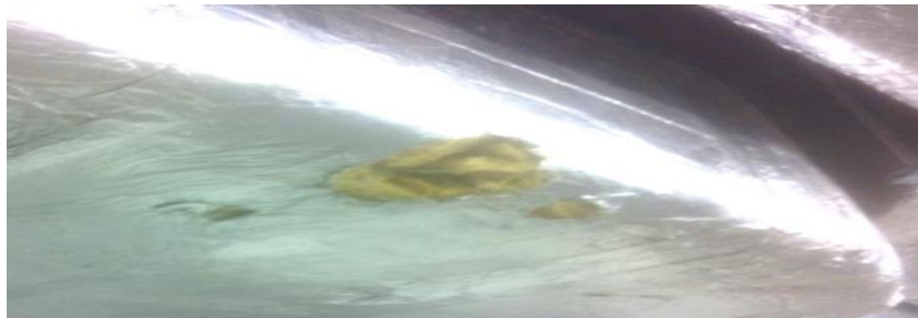
Figure 8. Damage of insulation at ventilation ducts as a result of fixation [6].
