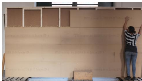
Figure 16. Application of wood fibre boards
