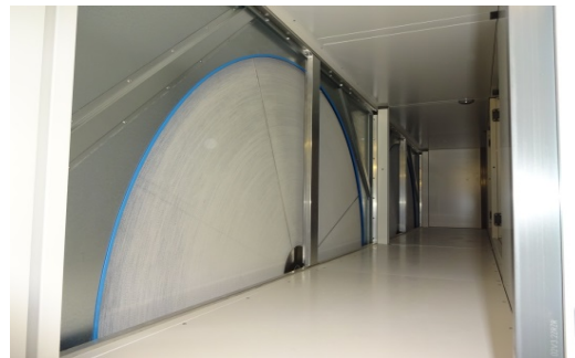
Figure 4: Rotation heat exchanger
