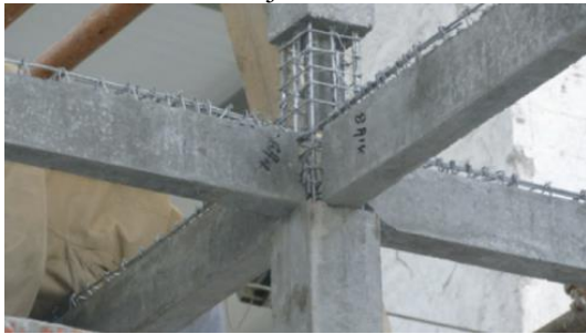
Figure 6. Erecting columns and beams.
