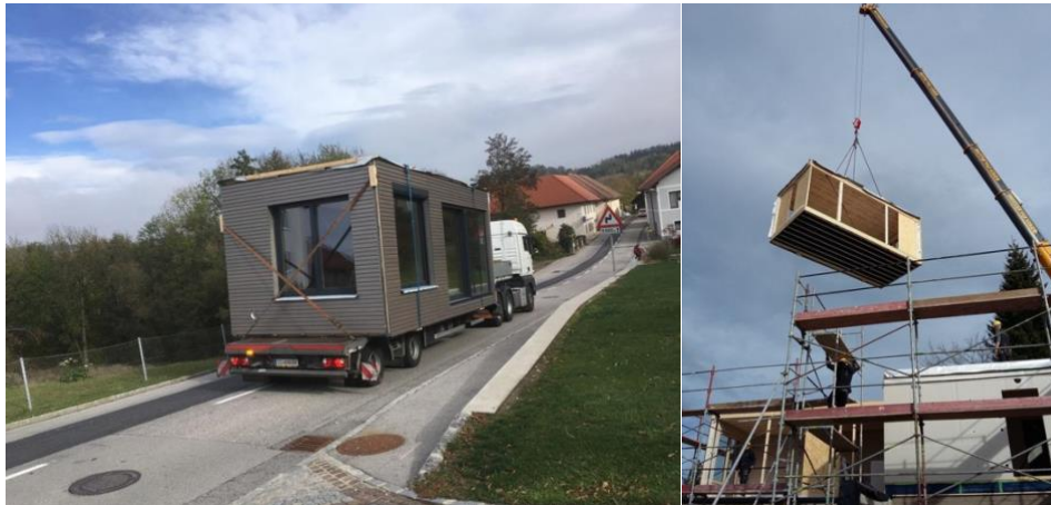
Figure 4. Transport and construction of a module based home [8]
